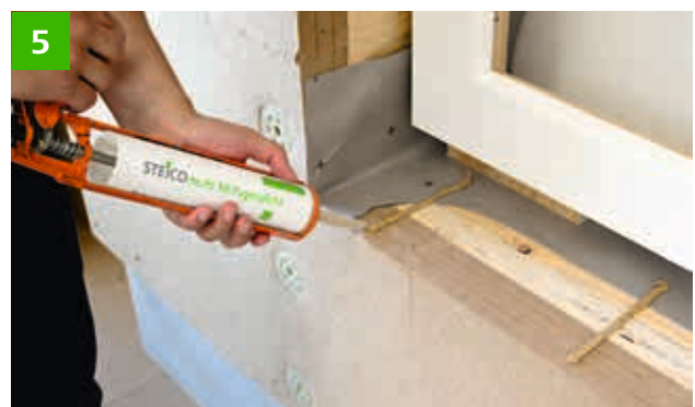
STEICOmulti fill adhesive beads are used to secure the insulation wedge against lifting off, e ≤ 30 cm.
