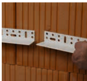
Attach angle rail
