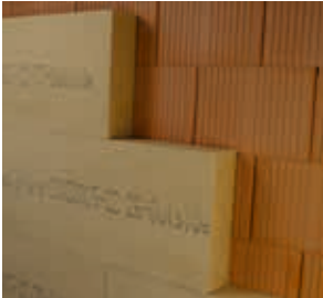
Installation of small-format square edge boards
