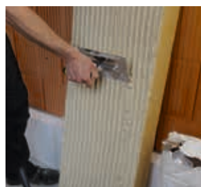
Glue the insulation board to a flat surface with full-surface bonding
